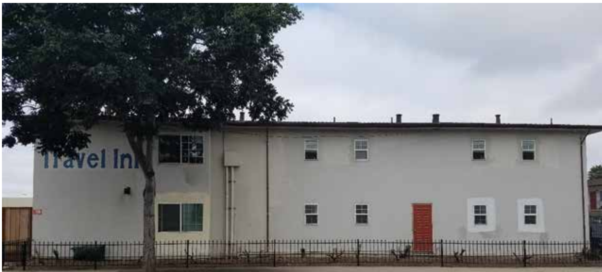
Permitted as an employee-housing facility, and inspected by HCD, the Travel Inn includes furnished rooms that meet the Employee Housing Act and the inn serves as home for workers in Salinas, California. (Photo credit: HCD Staff)
