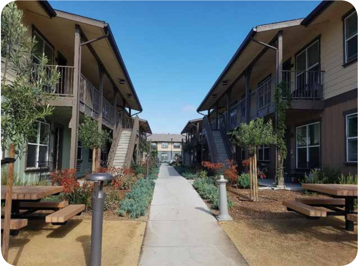
Located in Speckles, California, Spreckles Crossing accommodates up to 800 employees in 100 two-bedroom, two-bathroom units. The multi-unit structure, owned and operated by Tanimura & Antle, is under Monterey County Health Department enforcement authority. (Photo credit: HCD Staff)
